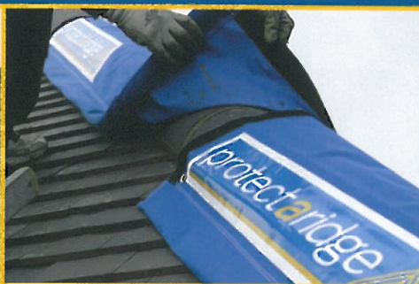
Laps secured by tough Velcro
