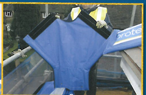
Special junction piece for mitred ridges
